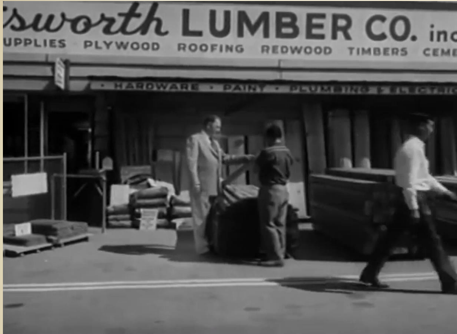
Ben Boydsten, Chatsworth Lumber northeast corner of Topanga and Marilla
