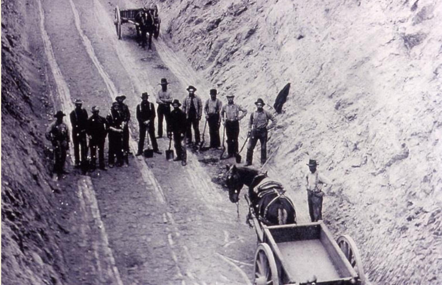
Grading crew posing for a photo in the Cut section
