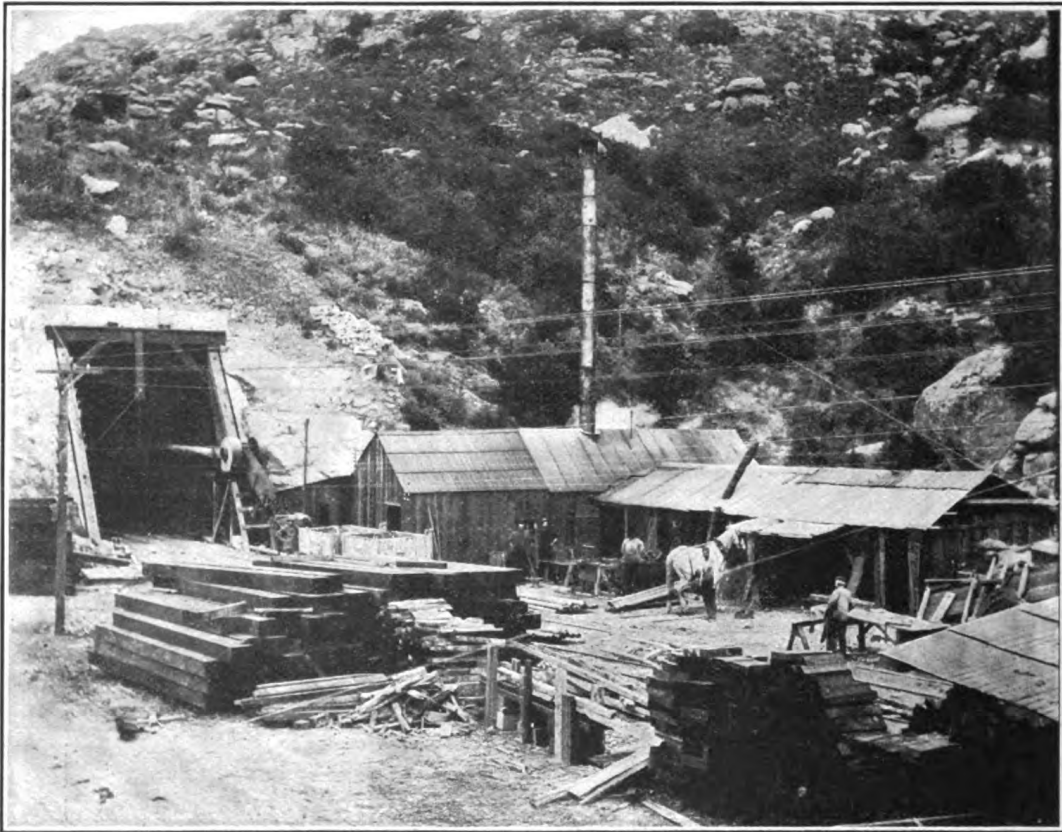
Soon . . . the train will hurry into and through the great opening which so lately was a part of Santa Susana's massive pile.
